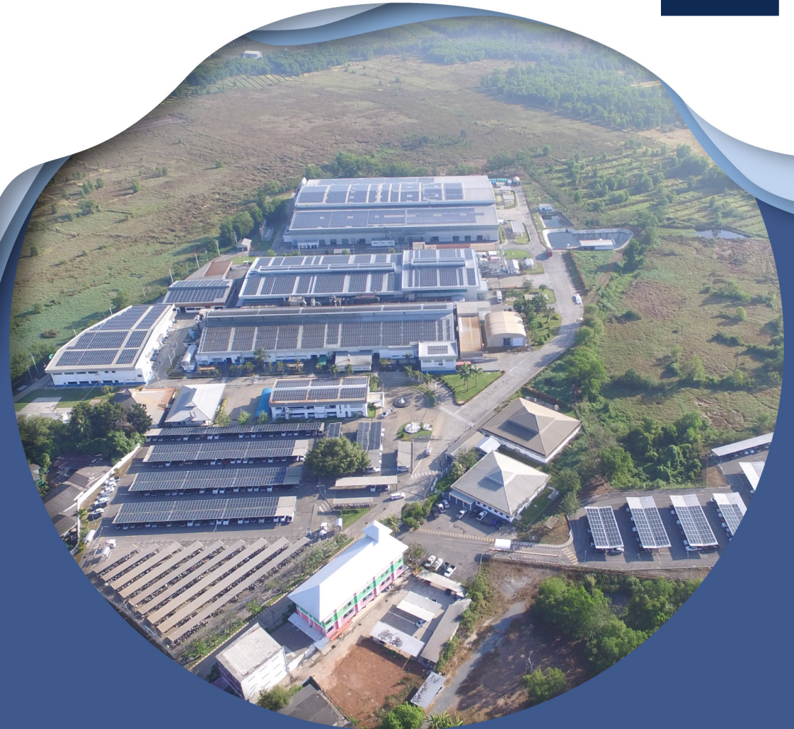
Graphic 23: solar panel plant Klaeng/Thailand
